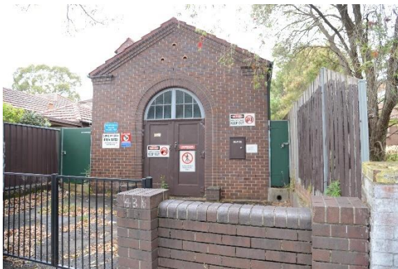
Figure 6.3 Heritage listed substation at 2B Cooper Street.
