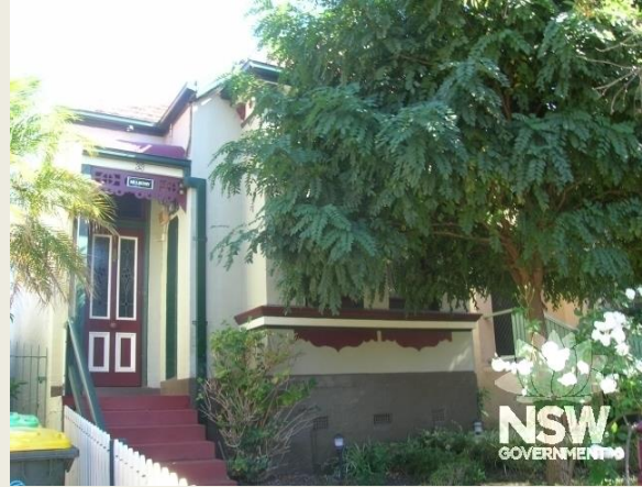
Figure 7.14 Primary elevation of 33 Wallace Street, Burwood, July 2020. (Source: NSW SHI)
