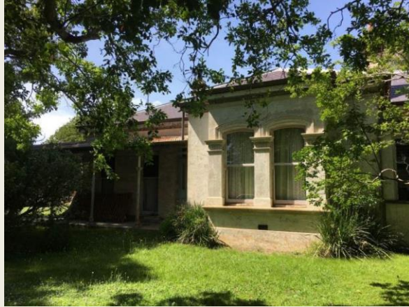
Figure 7.1 Northern elevation of 2 Cooper Street. (Source: Urbis 2021)
