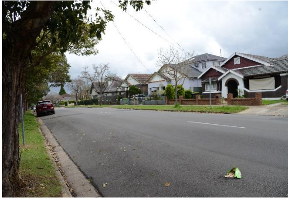
Figure 6.1 The Cooper Street context, showing the properties opposite the subject sites.
