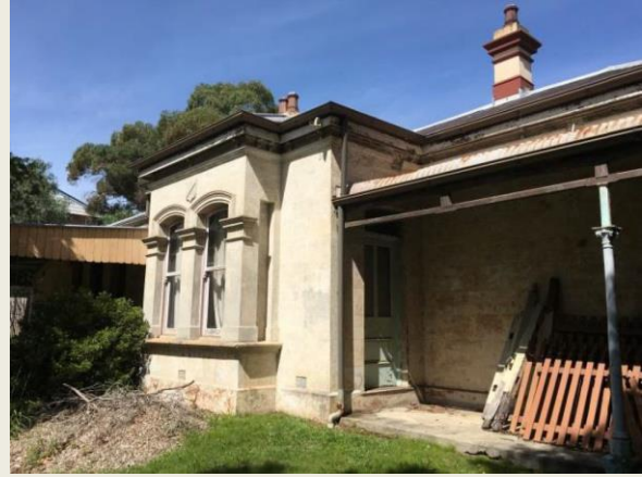
Figure 7.2 Northern elevation of 2 Cooper Street. (Source: Urbis 2021)
